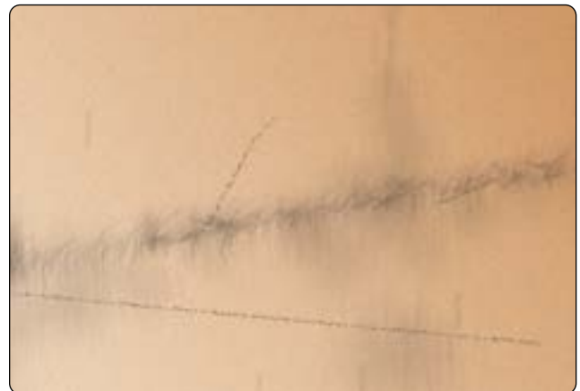
Figure 8-19. Example of sanding scratches.
