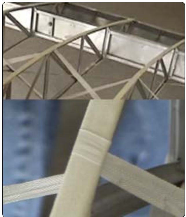
Figure 3-19. Inter-rib bracing holds the ribs in place during the re-covering process.
