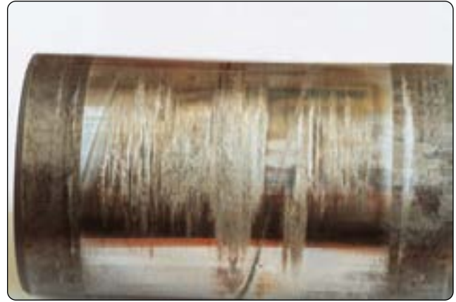
Figure 13-65. Galling is caused by rubbing of mating surfaces. The metal gets so hot it welds, and the surface metal is destroyed as the motion continues and pulls the metal apart in the direction of motion.
