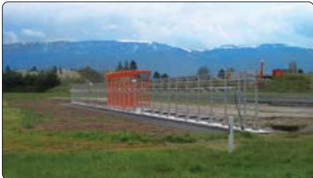
Figure 11-111. An ILS localizer antenna.
