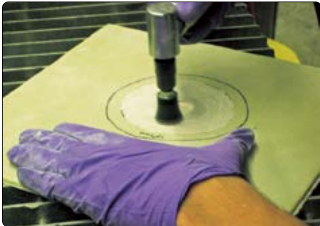
Figure 7-58. Taper sanding of repair area.
