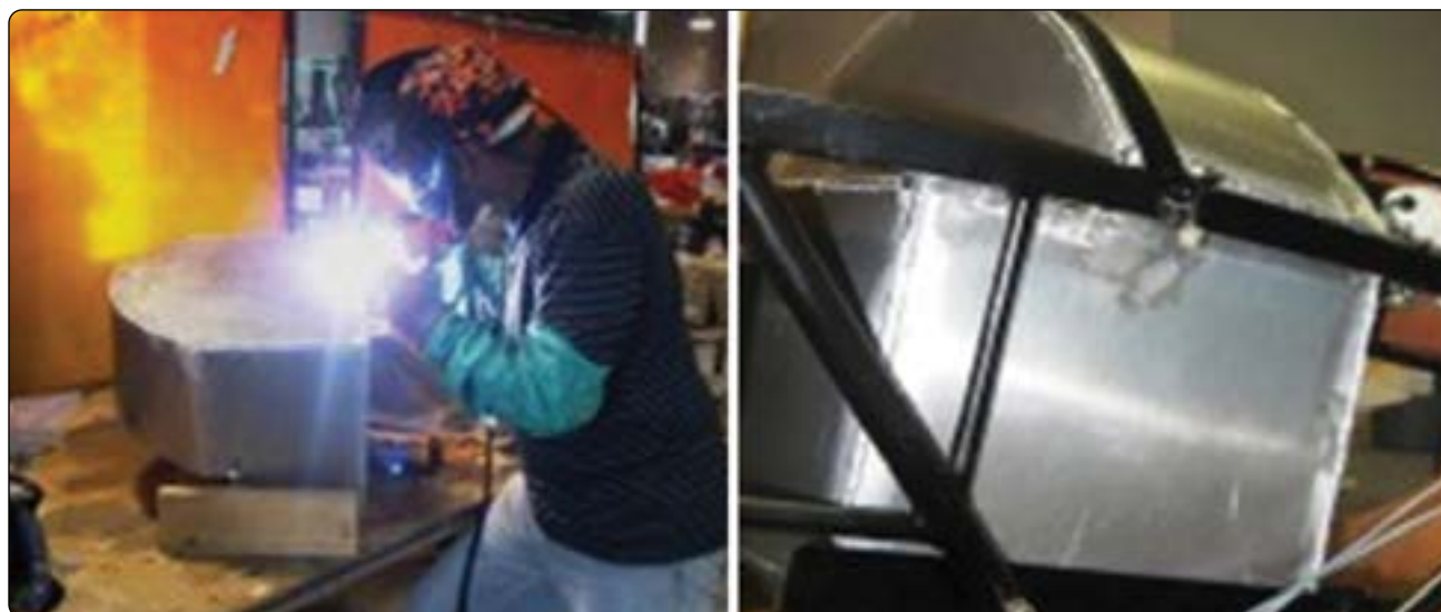
Figure 14-90. A rigid removable fuel tank with welded seams is repaired by welding.
