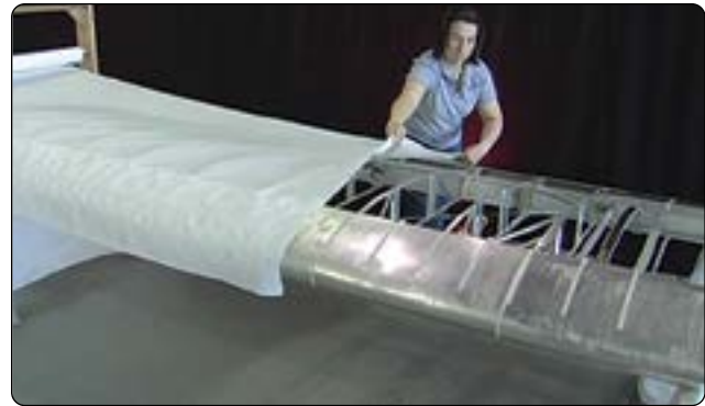
Figure 3-12. Laying out fabric during a blanket method re-covering job.
