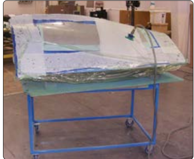
Figure 7-52. Envelope bagging of repair.
