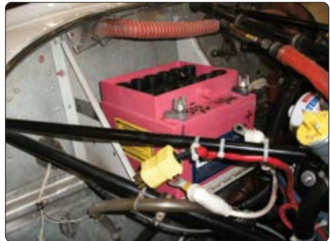
Figure 9-32. Lead-acid battery installation.
