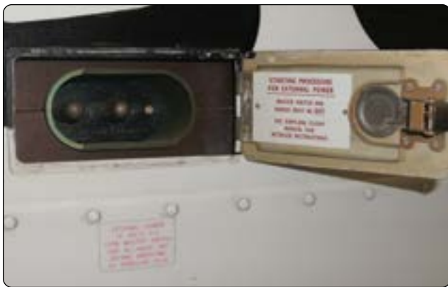
Figure 9-89. External power receptacle.
